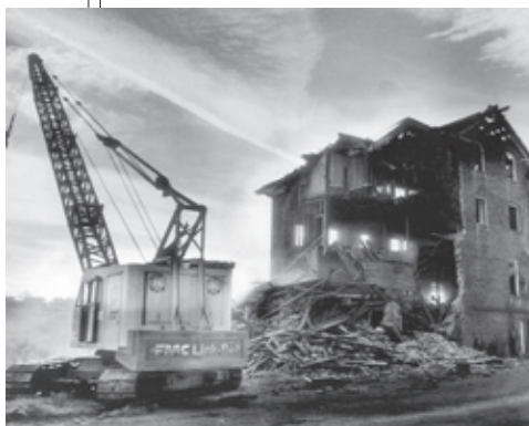
Demolition of the Christiansburg Institute campus
